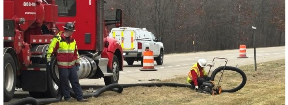
Contractors using manipulated lawn mowers to vacuum up plastic pellets on the side of the highway.
