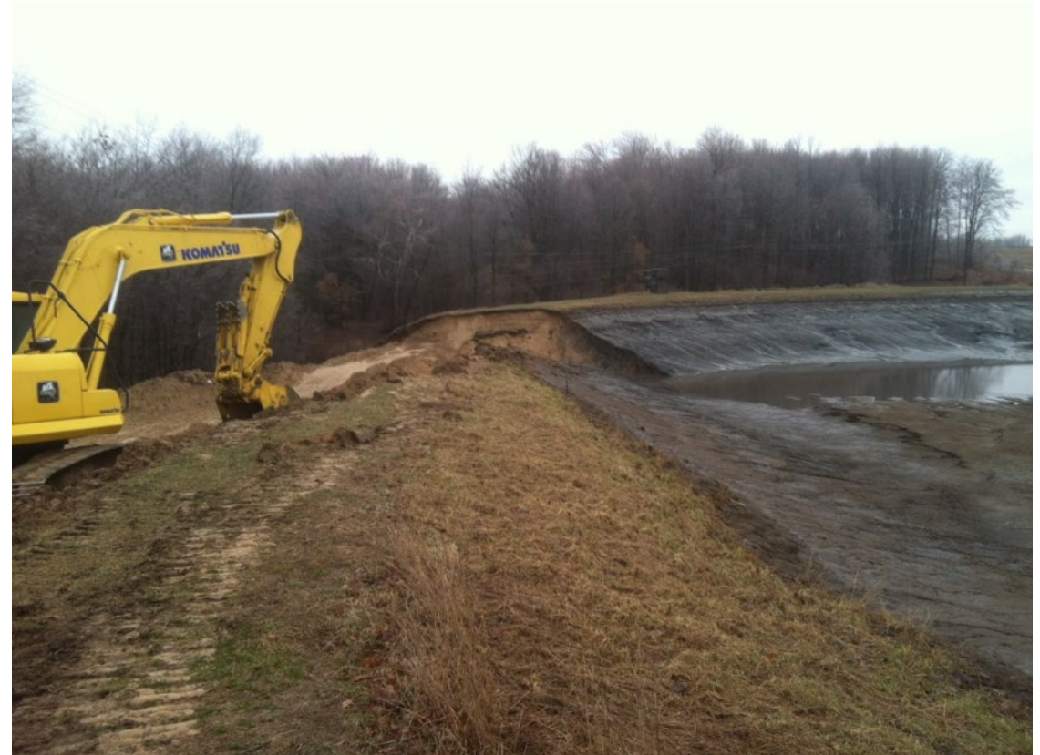
Open air waste storage structure failure.
