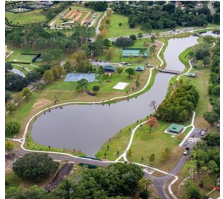
Lawne Lake Stormwater Reuse Facility Courtesy of Orange County, FL
