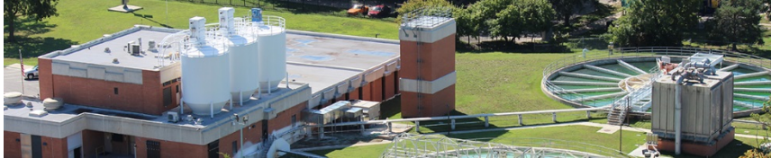
Manhattan Kansas Wastewater Treatment Plant Manhattan Kansas Population: 54,852 Median Household Income: $50,065
