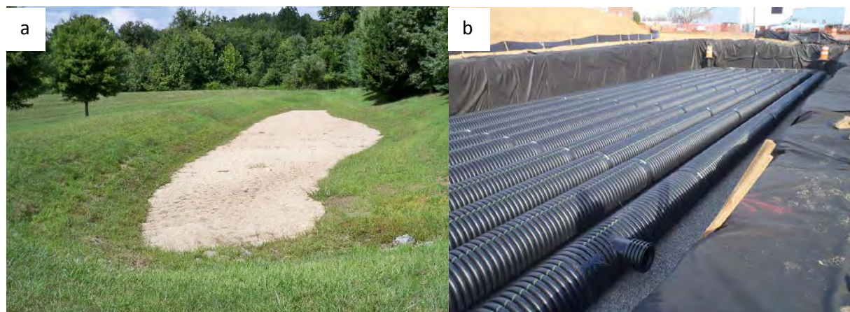
FIGURE 4-1 Aboveground (a) and belowground (b) stormwater retention facilities with infiltration. SOURCES: (a) Montgomery County Department of Environmental Protection; (b) Philadelphia Water Department.
