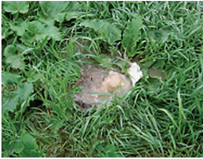
Figure 9. Water gushing from blowout
