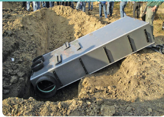
Figure 4: Water level control structure for tile drains.
