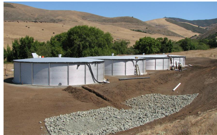
Rainwater catchment project near Pennington Creek, California, installed in partnership with the Morro Bay National Estuary Program, stores up to 296,000 gallons of rainwater for cattle troughs in the dry season.
