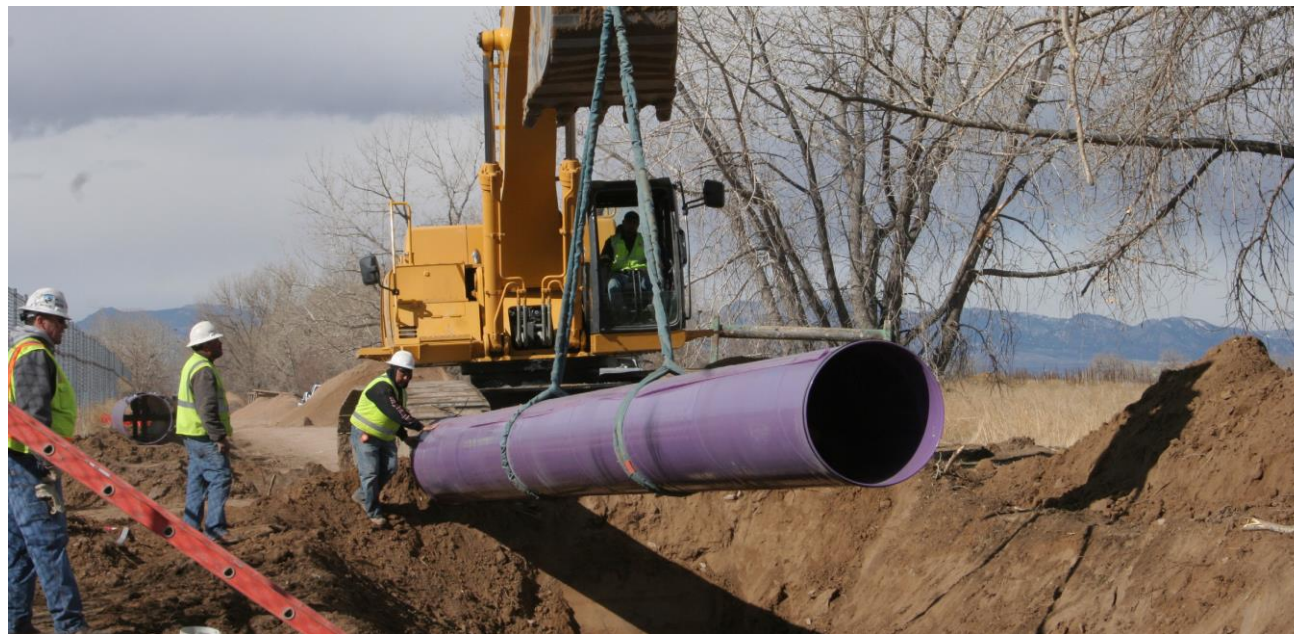
Denver Water contractors install a purple pipe used to deliver recycled water in northeast Denver, Colorado
