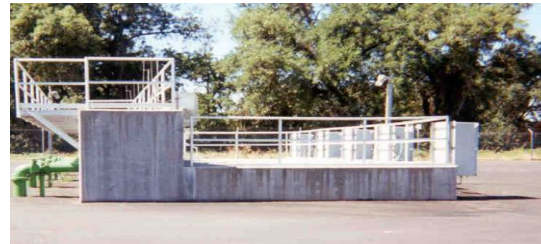
Continuous backwash filter – Lone, CA
