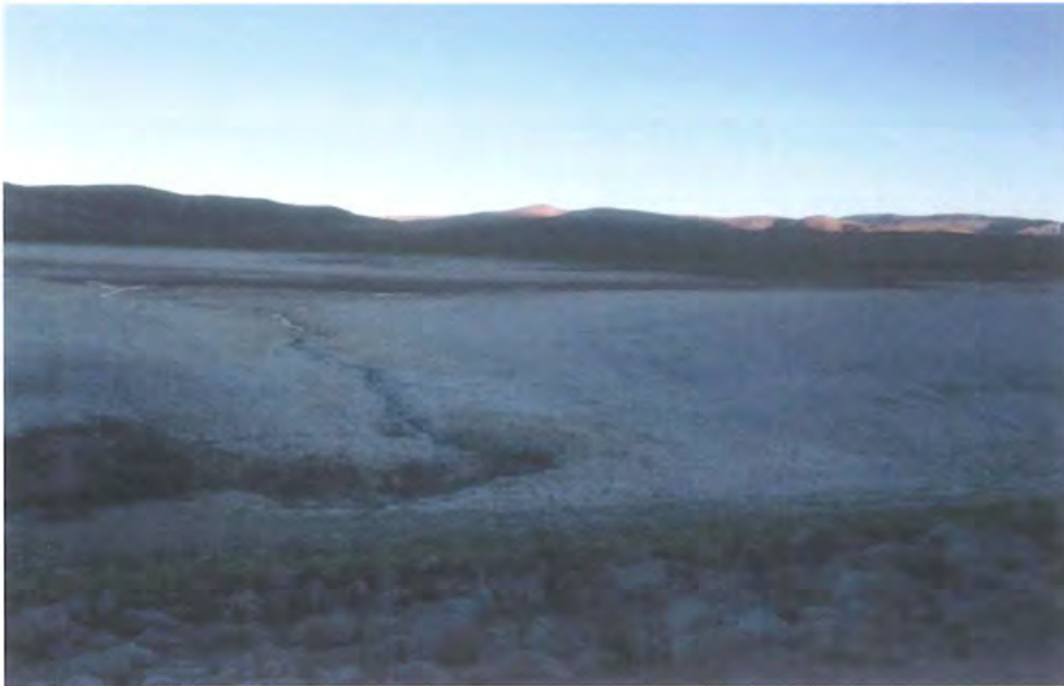
Exhibit A 9 Mile Irrigation Reservoir
