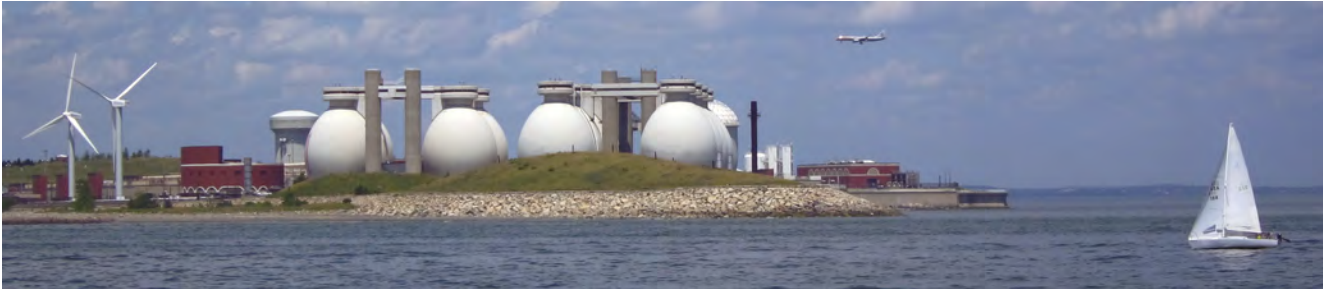
Deer Island Wastewater Treatment Plant, MA. Courtesy of Kirk Tracy, ACWA.
